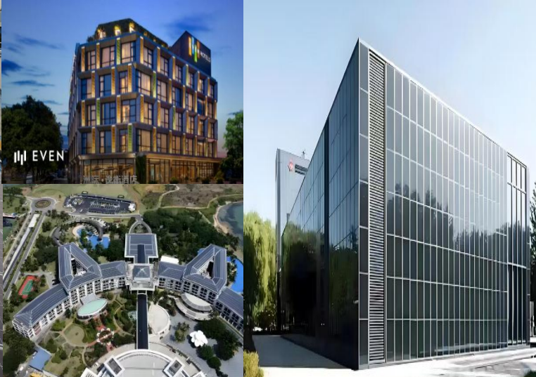
BIPV (Building Integrated Photovoltaic)
