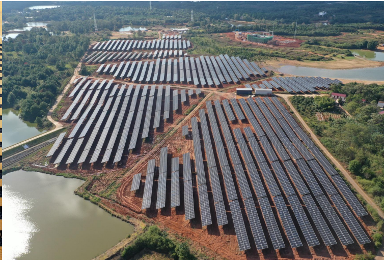
Forestry Power Plant
